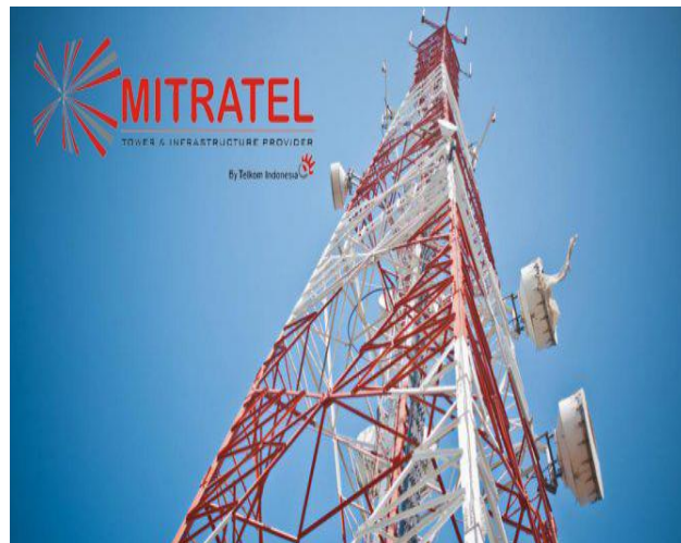
Gambar 2.1 Tower Transmisi PT. Mitratel [3]
